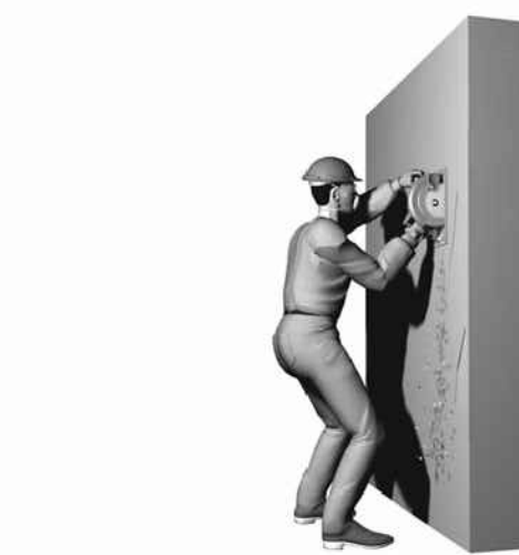
Fig. 3—Edge conditioning.
