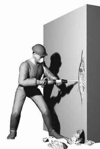
Fig. 2—Bulk concrete removal.
