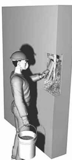
Fig. 8—Hand application of repair material.
